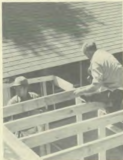
Frank Kowalski and Robert Hoover, from the Kingston church, construct a new support system for the roof.
