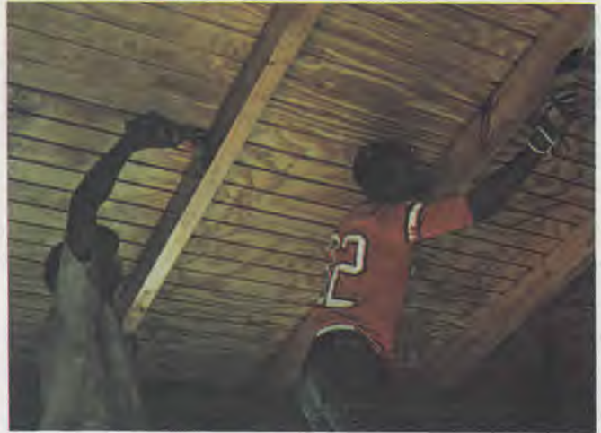
Students varnish ceiling of school.
