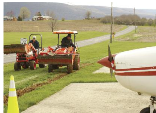
Volunteers fill settled trenches that cover wiring for the new landing lights.
