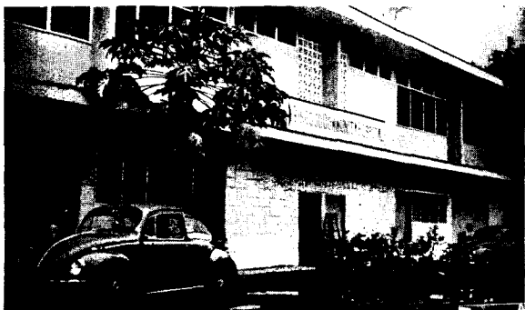
BRAND NEW: The Gingoog Community Hospital, a medical institution operated by the church, has just recently moved to its new location in the Cabuyo-an subdivision of Gingoog City. The building and lot cost Ps. 52,000.
