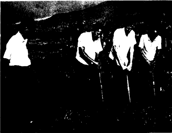
GROUND BREAKING. Two dormitories are presently under construction at Naga View Academy. Breaking the ground are V. N. Napod, Southern Luzon Mission president; O. C. Edwards, Philippine Union College president, and S. N. Napod, Naga View Academy business manager. M. G. Jereos, left, North Philippine Union secretary, looks on.
