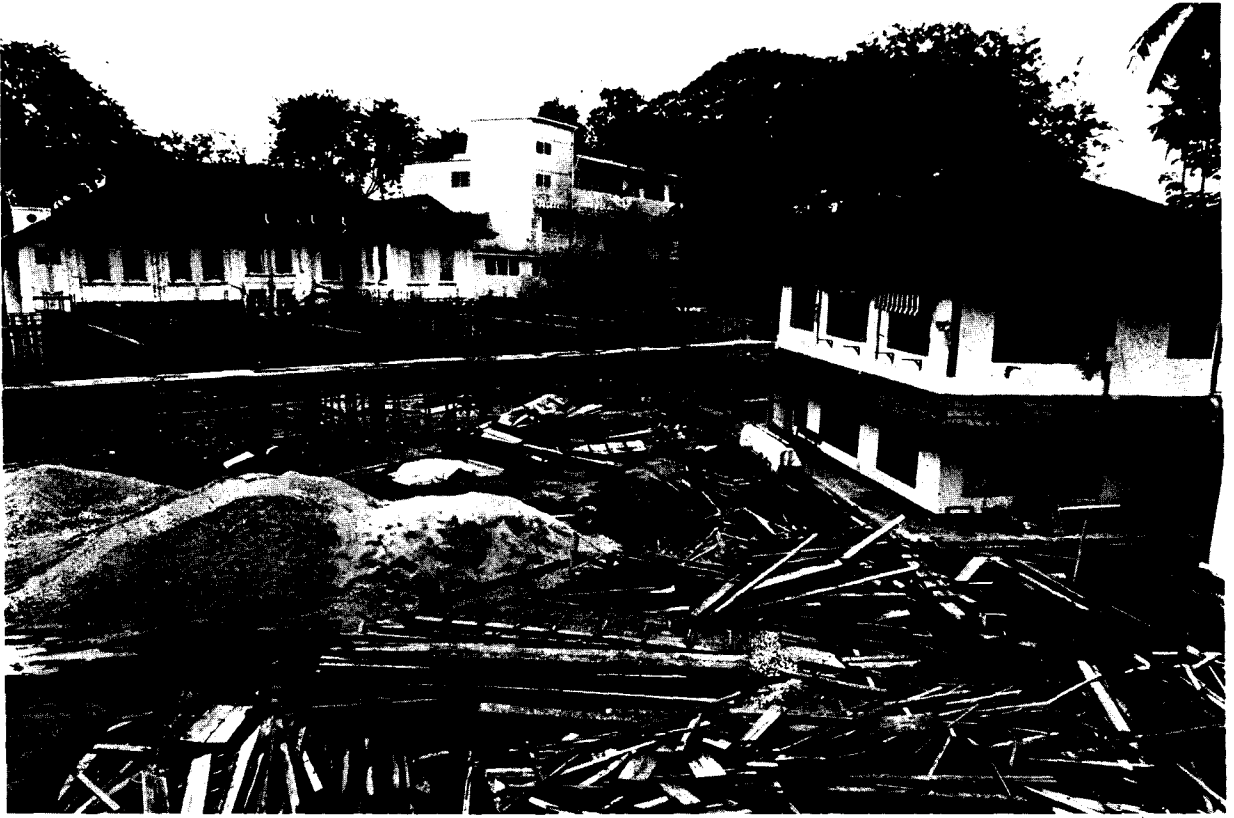
This is the way it looked in August. The US$182,000 addition to the Penang Adventist Hospital is expected to be completed March 1, 1974. The addition will increase the patient bed count by 19, bringing it to 135 beds.
