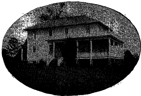
Oakwood Sanitarium, (Colored) Huntsville, Alabama
