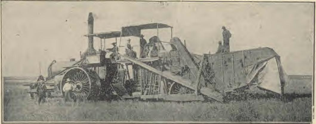
A GRAIN HARVESTER : CUTS, THRESHES, AND SACKS GRAIN IN ONE OPERATION
