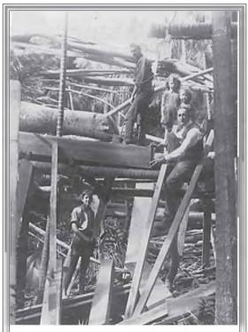
A primitive sawmill. One man on top & another underneath to operate the pitsaw. Arthur Ferris pushing the logs across the saw. Edna & Muriel are standing behing their father.
