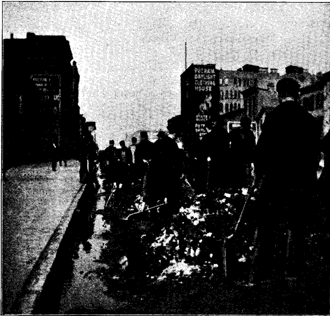
MEN AT WORK ON THE STREET
