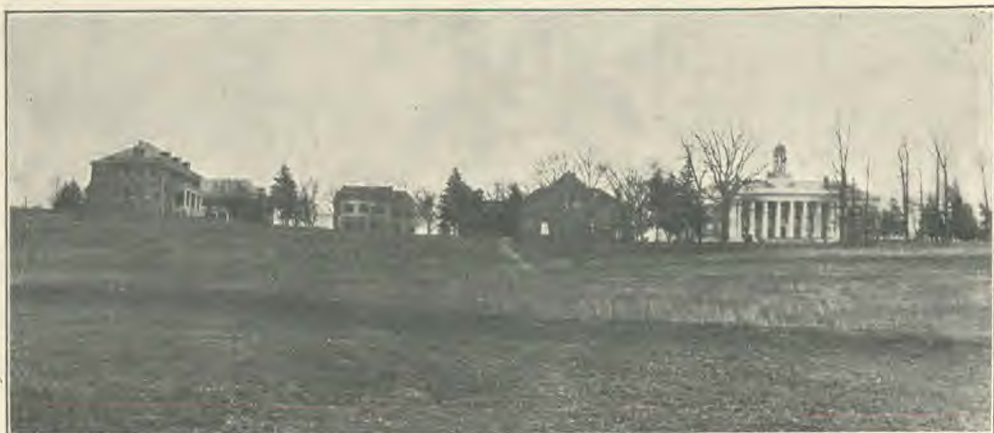
PARTIAL VIEW OF BUILDINGS FROM FRONT
