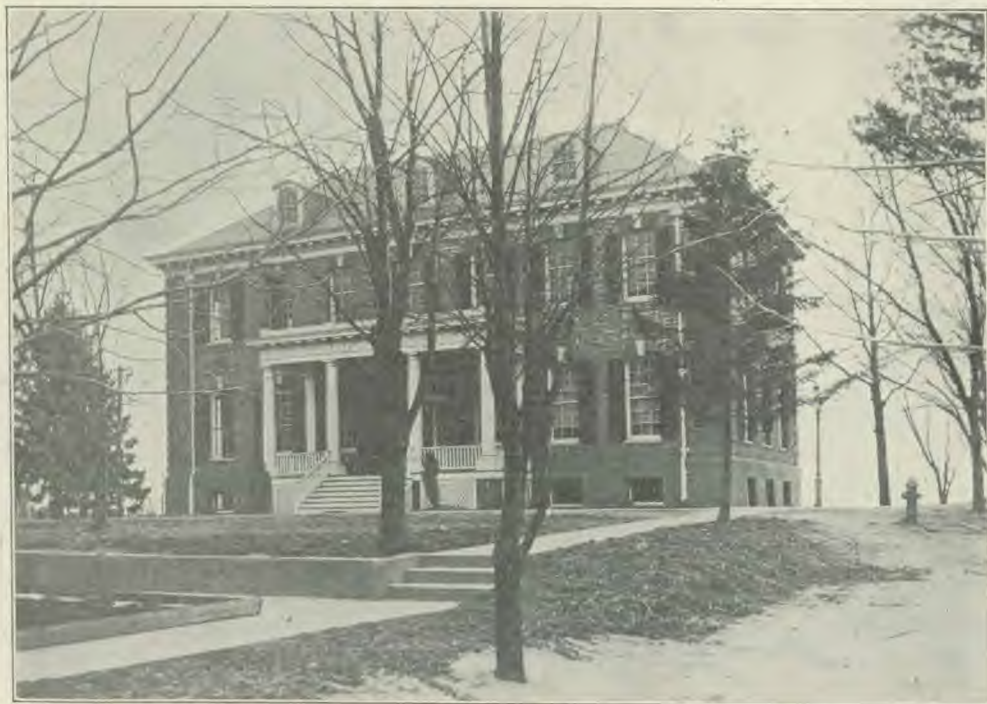
ONE OF THE COTTAGE HOMES BUILT BY THE BOYS
