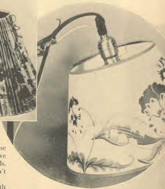
Upper Left: Frayed Cord on Electric Iron Should Be Immediately Repaired or Replaced if in Too Bad Condition. Middle: Wire Is Exposed, and the Cap on Socket Has Become Loosened. Don't Permit Such Things to Occur in Your Home. Above: Note a Properly Wired Lamp
