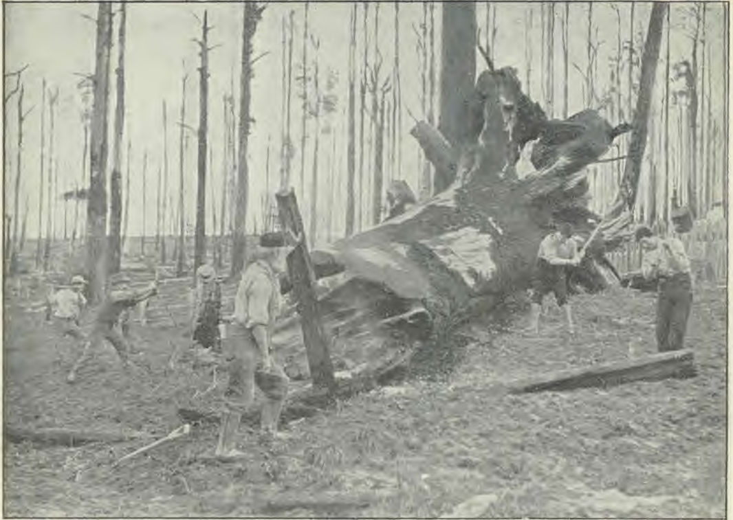
CLEARING THE LAND
