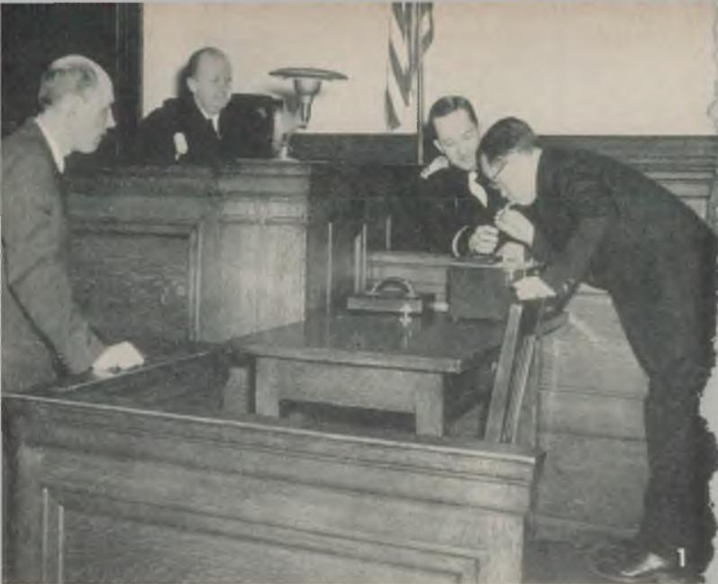
1. As judge and attorney watch, Borkenstein, in uniform, gives a Breathalyzer test in court. This hearing was part of a program done before TV cameras at Chicago. An automatic release allows all air to escape from the cylinder except the last 100 centimeters needed for the test. Thus, surface air is "blown off" so deep lung air, not throat air, is trapped. A drinking man wastes his time if he tries to beat the test.
