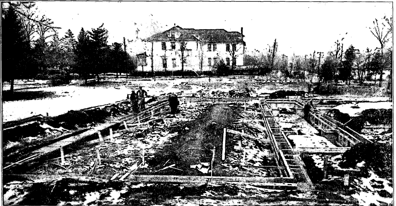
FOUNDATION FOR LIBRARY IS NOW COMPLETE
