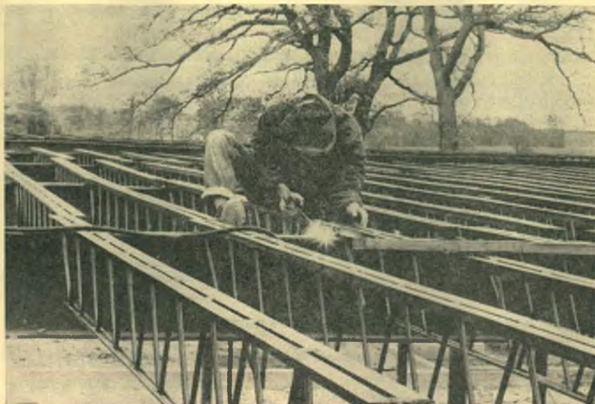
Bill McDonough, a senior student, is putting his welding training to good use as he is welding steel bar-joint in the new administration building.
