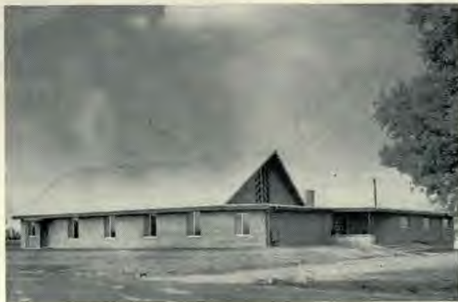
The new Lapeer Church has a good location along a busy highway and is a blessing to the congregation as well as a good addition to the city.
