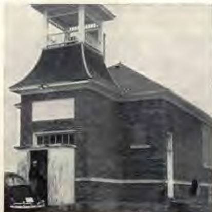
The Clear Lake congregation recently bought this birch school house for their church school. On October 8 they broke ground for a new addition.
