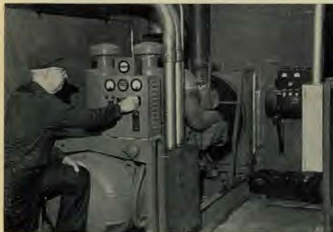
Ross Henderson checks out the hospital's powerful deisel generator which is capable of producing enough power to keep the institution going on an emergency basis in the event of a power failure.
