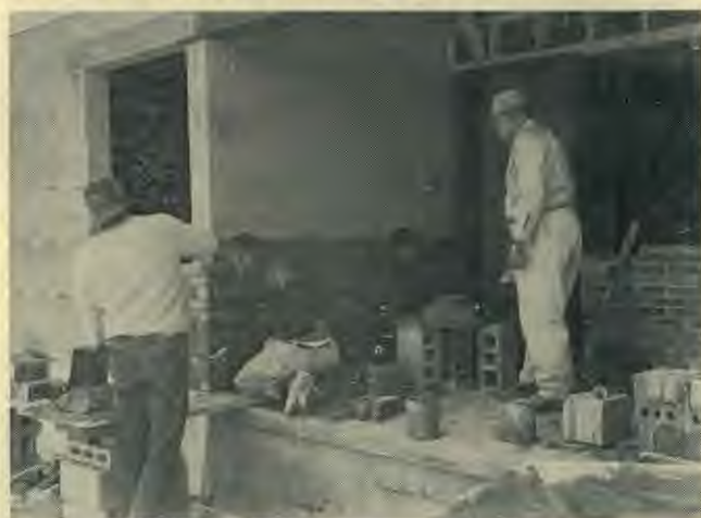
The masonry crew installed the last small section of brick on the exterior of the dormitory at the same time the concrete roofing was put into place.
