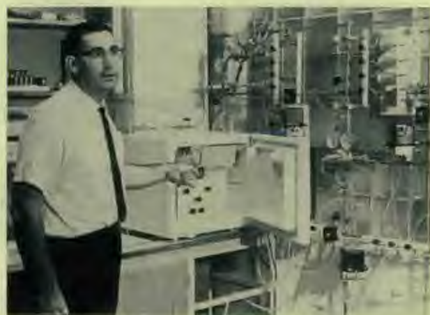
Dr. Leonard Hare, associate professor of biology, points out features of his home-built amino acid analyzer he will use for research in the chemistry of flowering.
