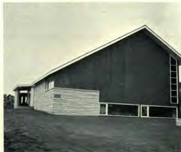
The Oakland church was recently remodeled.
