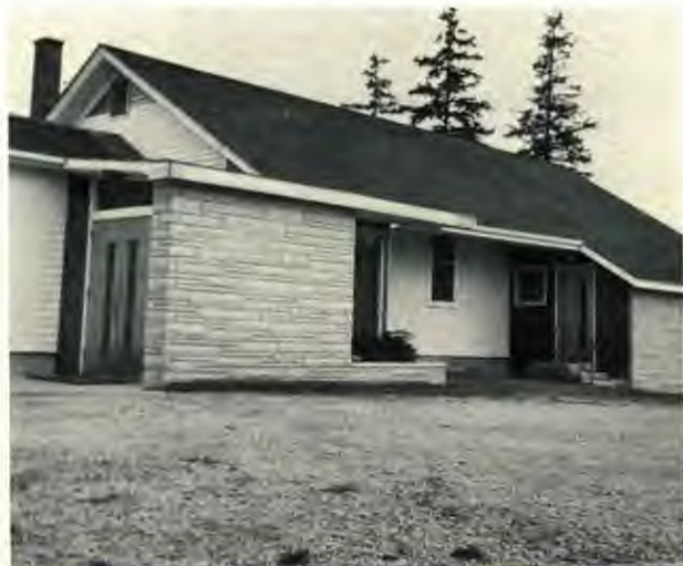
The rear of the Oakland church shows part of the old building. Adventists have worshiped here for 105 years.
