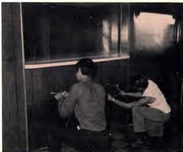
Leslie McKinney and David Johnson put finishing touches on remodeling of the monitors' station at Indiana Academy.
