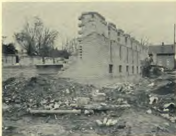
The shell of the new Pointiac Southside church takes shape.
