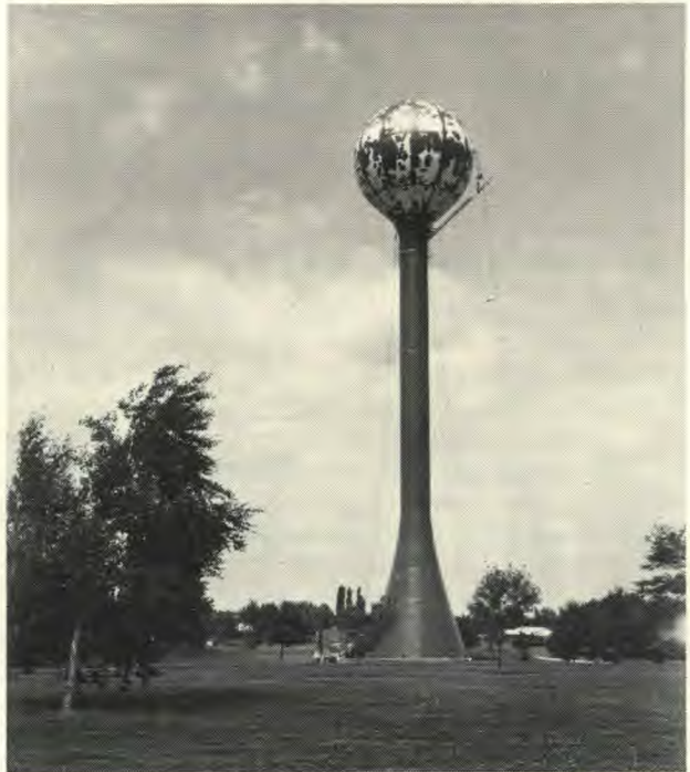
A familiar landmark at B.V.A. being refurbished.
