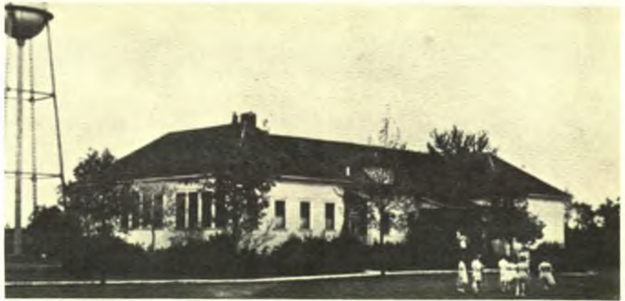
The old academy building
