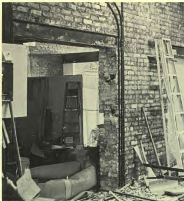
Workmen removing the plaster from the wall dividing the building discovered arches that had been built into the wall in just the right places nearly sixty years earlier.
