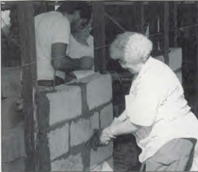
In the foreground Doris Evans, a church member from Eagle River, WI, works on a block wall of the new church in Santiago, Dominican Republic. Most of the 19 Lake Union volunteers were from Wisconsin.
