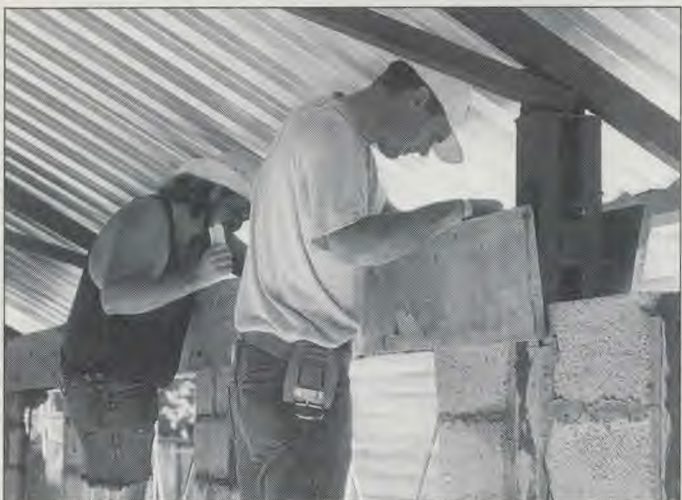
From left, Travis Simpson, Climax, Michigan; and Bob Slikkers, Holland, Michigan; form up the bond beams that hold the walls together at the top.
