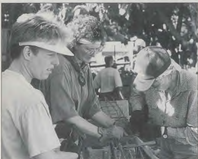
From left, Colleen Asmussen, Madison, Wisconsin; Barbara Szaflarski, Coon Rapids, Minnesota; and Lucille Sayen, Trenary, Michigan; tie the reinforcing steel rods for the bond beams.
