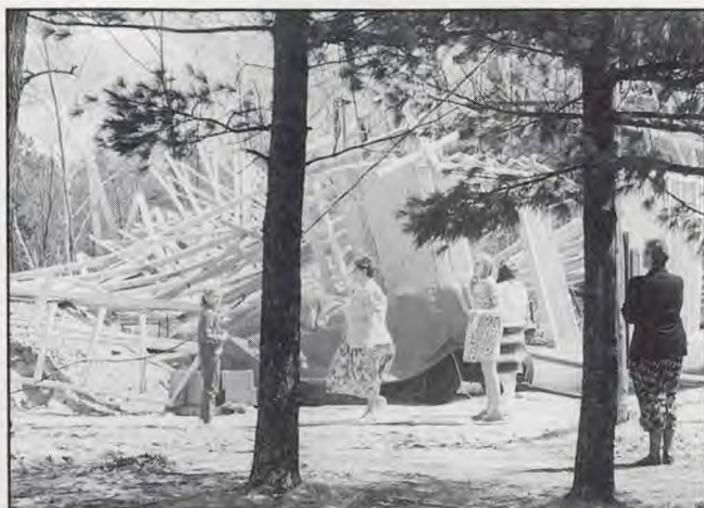
A windstorm reduced the roof trusses of the new lodge to a "pile of matchsticks." Volunteers are needed to help clean up and rebuild.
