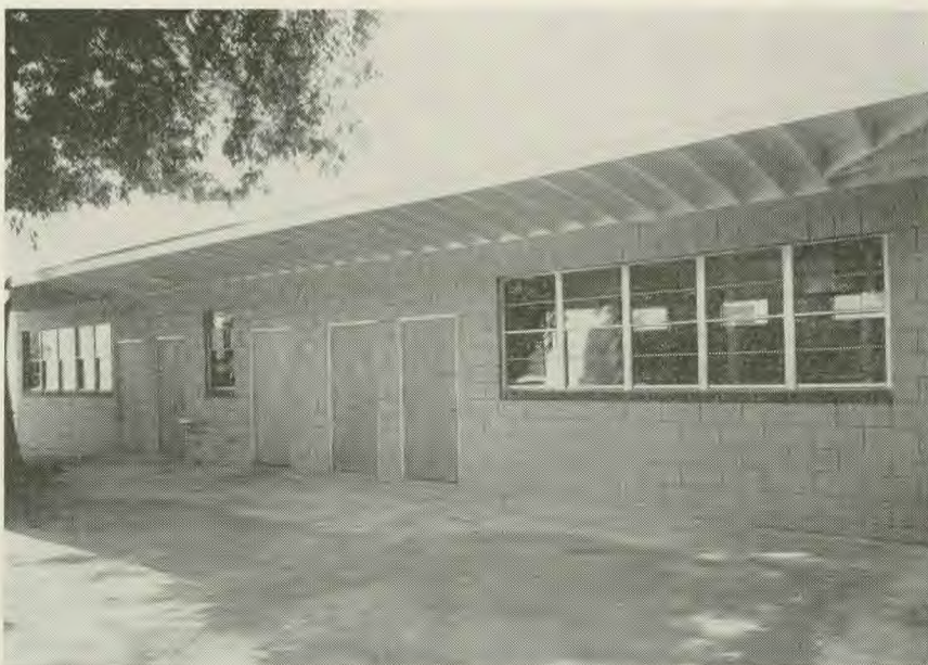
Baton Rouge school annex.
