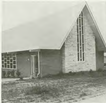
The new Shepherd Drive SDA church in Columbus, Georgia, is fully air conditioned. It seats 350 and is valued at $100,000. Earl J. Lewis, pastor, supervised the construction.
