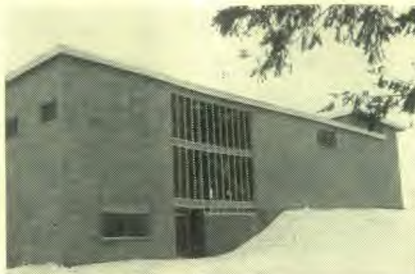
New Music Building nearing completion.
