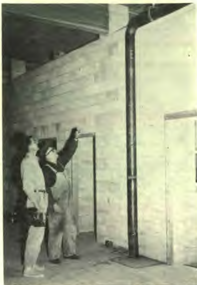
Bill Greenley, Industrial Arts instructor, and Don Lutts, maintenance supervisor, examine low pressure steam line that will carry steam to the fresh air heaters at U.C.A.
