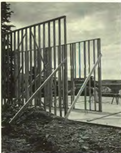
Off to a good start on the new Juneau Church School.
