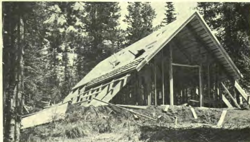
Museum under construction at Big Lake Youth Camp.
