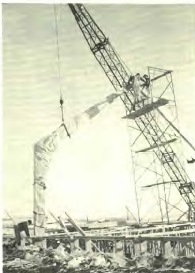
The strong arm of the crane gently nudges the first church beams into position.
