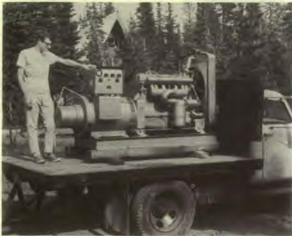
Jim Robertson, summer intern with the Oregon Conference, examines the new generator plant ready to be unloaded at Big Lake Youth Camp.
