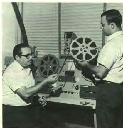
Film inspection is a vital part of processing as films are sent out across the United States to TV stations. Each time a film comes back it is run through a machine that checks the film carefully for scratches, breaks, or other problems. Checking over films are Ray Bryant and Fred Figueroa.
