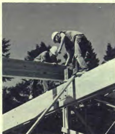
It takes some tricky balancing as Glenn Zollinger and Don Loren guide the laminated beams being swung into place by a large crane.
