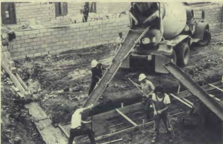
Two days after block laying began, four volunteers work feverishly to get the rest of the footings poured before the block layers catch up.
