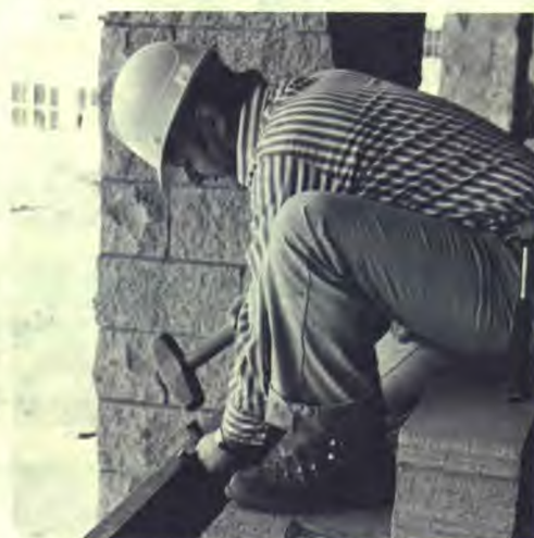
Volunteer Clifford Sorensen chips away cement to install a bolt.
