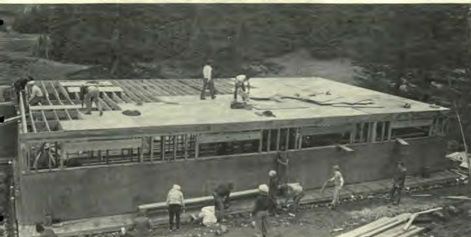
The structure starts up on the first day following completion of the foundation.
