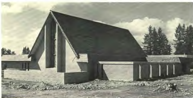
Newly completed Enumclaw Church
