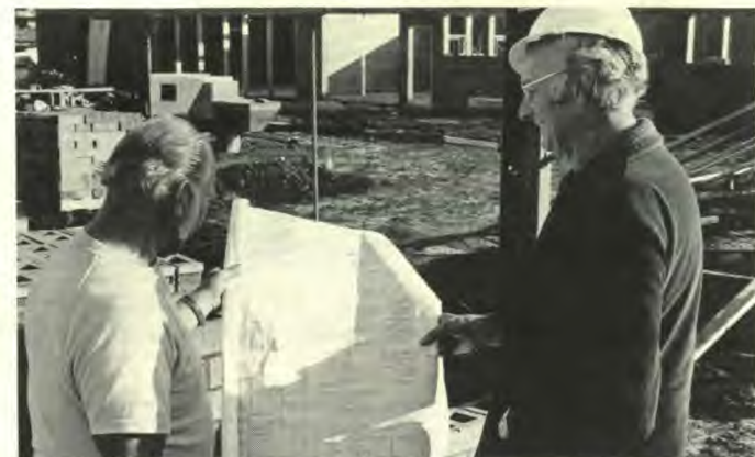
Masonry contractor Leon Bock and job superintendent Foster Campbell commented that additional bricklayers are needed for the Walla Walla General Hospital project.
