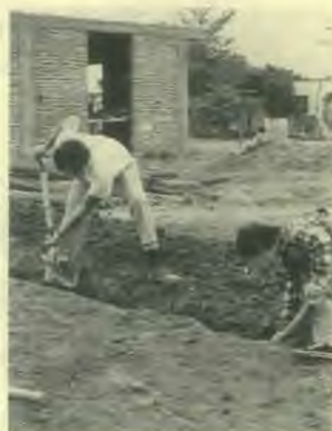
The fellows spent many hours digging trenches in the hard clay soil to bury electrical wires.
