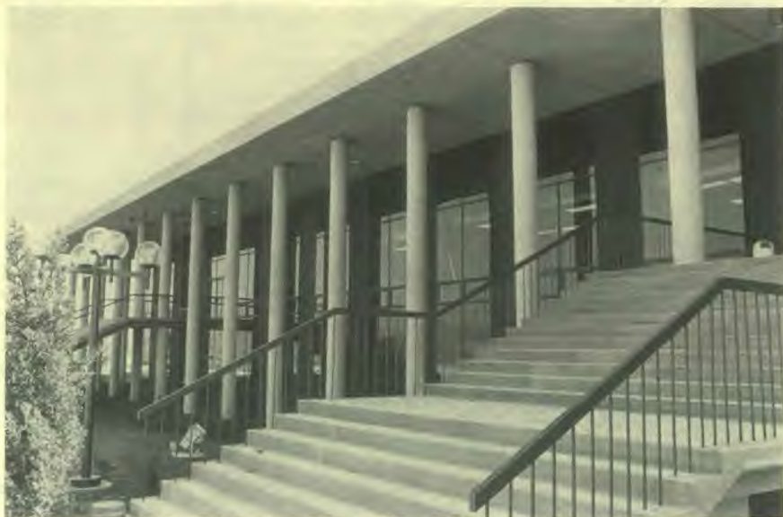
The SDA Radio, TV and Film Center in Thousand Oaks, Calif., is the new home of Faith for Today. Here the telecast currently shares common service and production facilities with "It Is Written" and "Breath of Life."
