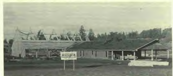
Harold Davis, a daily workman, sharpens his saw (above left); Ed Bauer, Linnea Balkan, Linda Bauer and Keith Brown laid shakes on the classroom section (above right) and the combined efforts of the members will soon result in a finished church.
