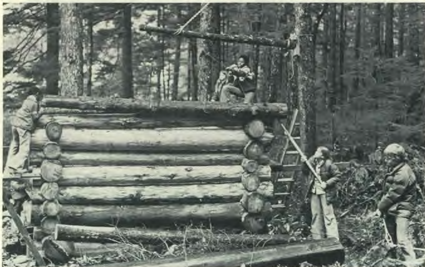
Juneau students discover the effectiveness of teamwork as logs are easily lifted and guided to the right place for scribing, notching and the final perfect fit.
