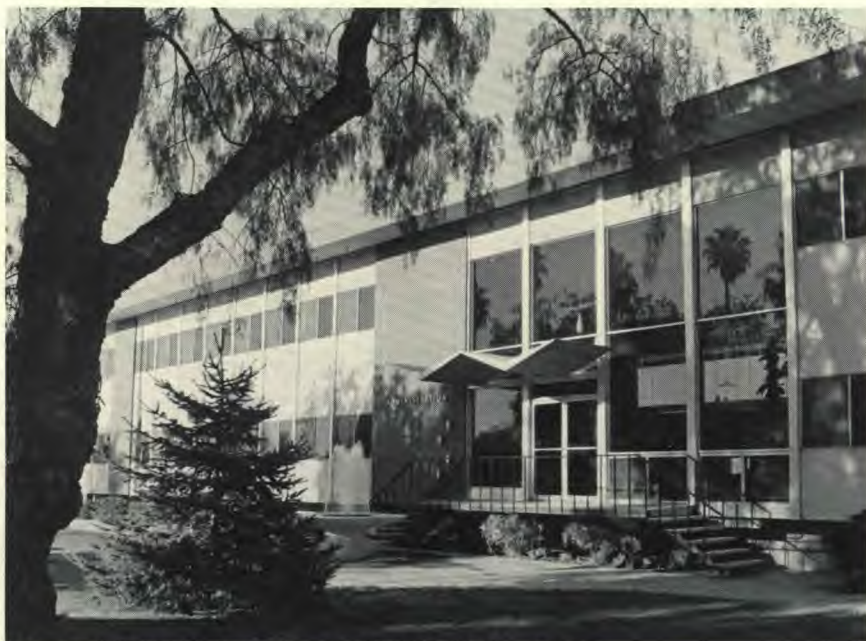
Hub of activities at the Pacific Press is the administration building.
