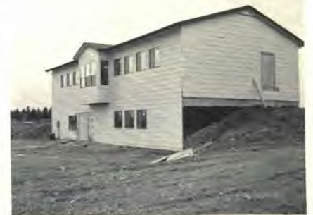
NEW SCHOOL COMPLETED. Students at Kalispell are enjoying the facilities of their new school. The building includes two classrooms, library and study area on the upper floor. The full basement on the lower level can be used by the school and church for various functions. It is hoped that the large acreage adjoining the school can be used for practical instruction in agriculture. The old school has served its purpose well but increased enrollment necessitated its retirement.
