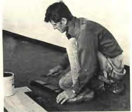
Floyd Reed, a stonemason and general handyman, proved to be an answer to prayer. At the time when a mason was desperately needed on the Industrial Arts building, he offered his services.
