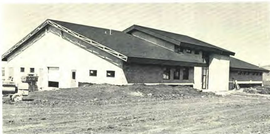
Newly completed Industrial Arts building at Mount Ellis Academy.
