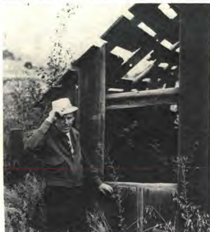
Frank Stiles stands by the woodshed which was built about the same time as the Fruitland Pioneer church. The church has been refurbished; the woodshed still tells the story of what the elements can do when a building stands unattended for 30 years.
