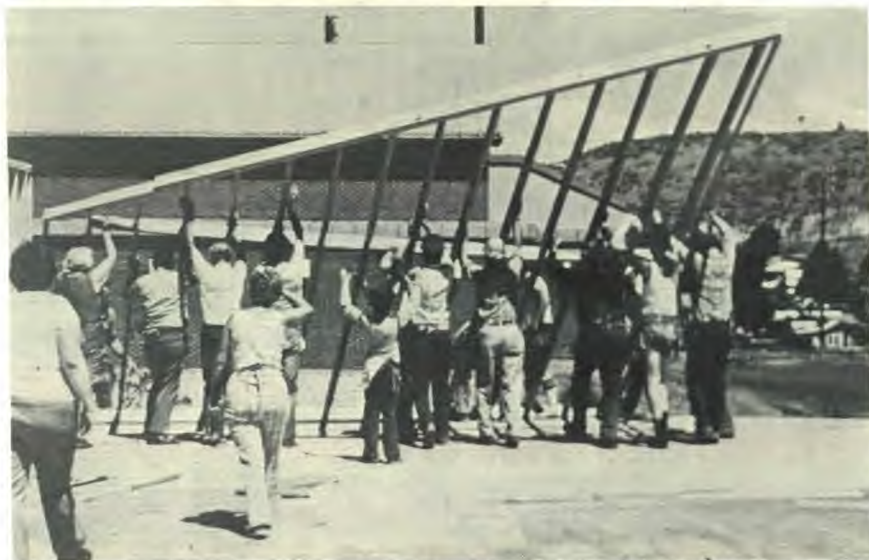
Maranatha Flights and Omak Church members raise the walls on the new structure.
