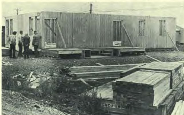
The church-parsonage in Kotzebue is built on a gravel "pad" which insulates the building from the permafrost a few inches below the topsoil.
