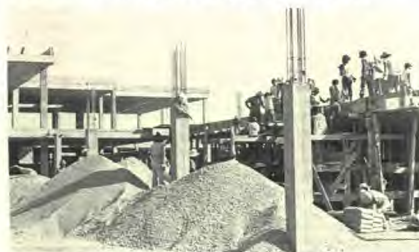
Construction view of new hospital building, August 1979.
