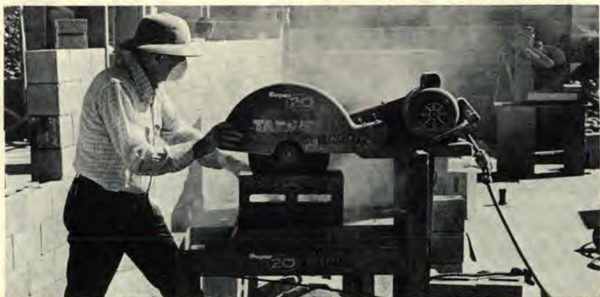
It's not the most glamorous job on construction, but someone has to cut concrete blocks. Orville Hamilton, Twin Falls, accepted this as one of his assignments.
