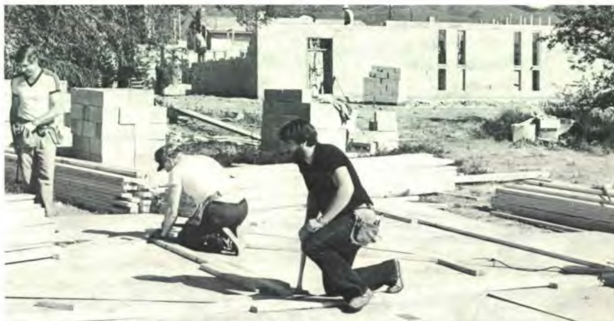
Volunteers assemble trusses while the concrete block school takes shape in the background.
