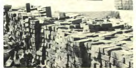
The lighter bricks are dirt and cement pressed under a ton of pressure. Each had to dry about two weeks, as they had to be watered frequently to prevent cracking.
