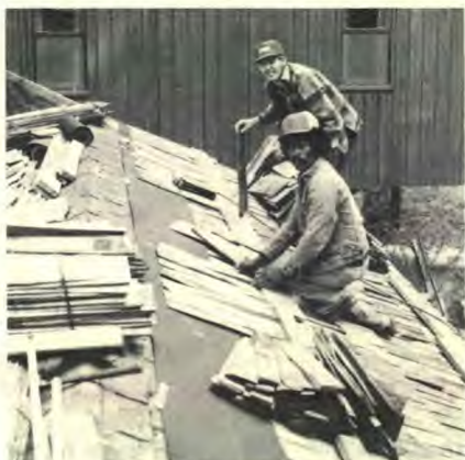
Techur Rengulbai from Palau and Ed Townsend apply shakes to the roof of one of the dormitories.
