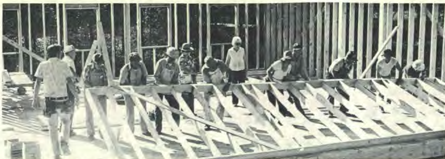
Newport Church members join with the Maranatha Flights taskforce to raise a major section of outside wall framing.
